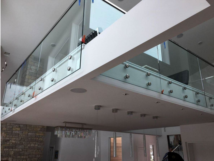
Glass Guard Rail: Stand-Off Mount Glass Application: Clear; 1/2" Tempered Glass (Required)
