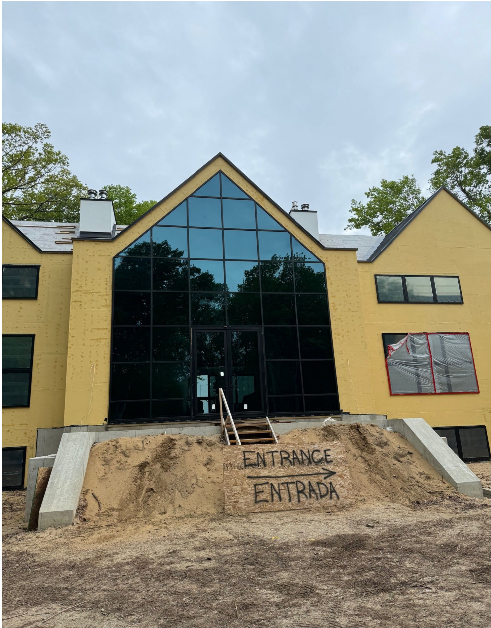
Exterior Application: Commercial Framing used to Create Dynamic Full Exterior Wall of Glass Glass Application: Insulated Glass Units; Tempered Glass (Required)
