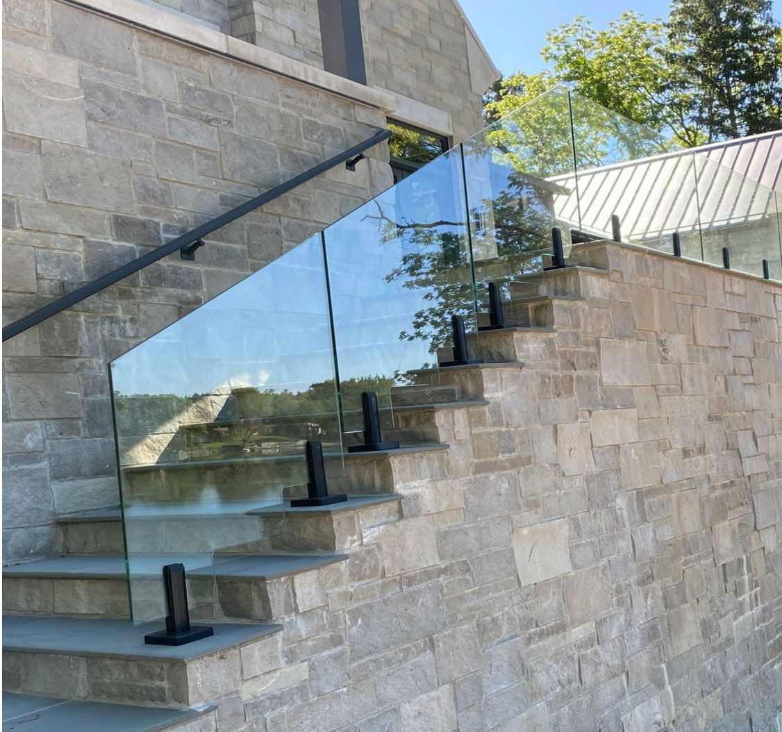
Stair/Wind Screen with Stanchion Mount Mechanism
