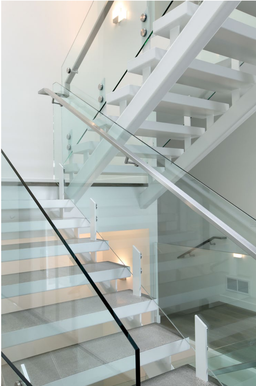
Custom Stair Rail: Steel Stanchion design and Stand-offs with Integrated Rail Glass Application: Clear; 1/2" Tempered Glass (Required)
