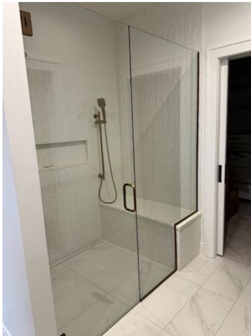
Euro Door/Panel Buttress Application (w U-Channel)
