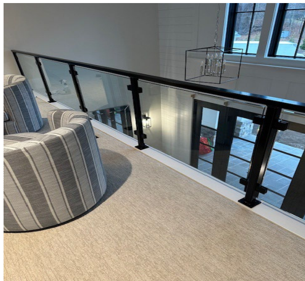
Glass Guard Rail: Z-Clamp Mount with Post/Top Cap Glass Application: Clear; 1/2" Tempered Glass (Required)
